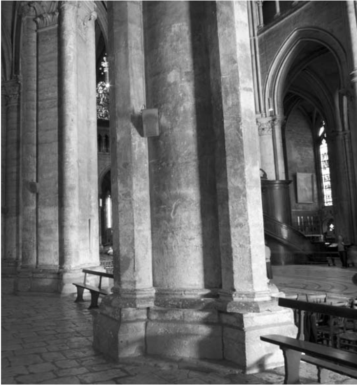
The pier cross-sections in the nave of Chartres alternate between circular and octagonal. Note that the four subsidiary columns in these compound piers have the opposite cross-section to the main columns. (Photo: Alex Rowbotham/AGRFoto.)
