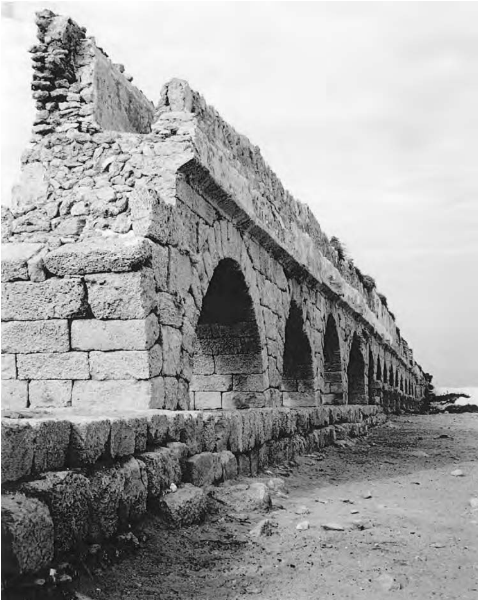
Aqueduct at Caesarea Maritima (B. Matlock)
