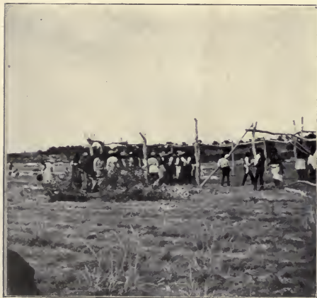
FIG. 44. Erecting the lodge.
