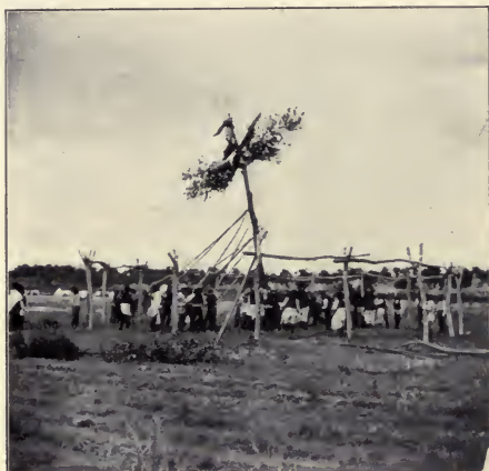
FIG. 54. Raising the center-pole.
