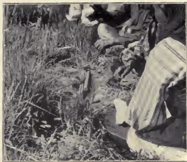
FIG. 19. The pipe-tampers and new earth.
