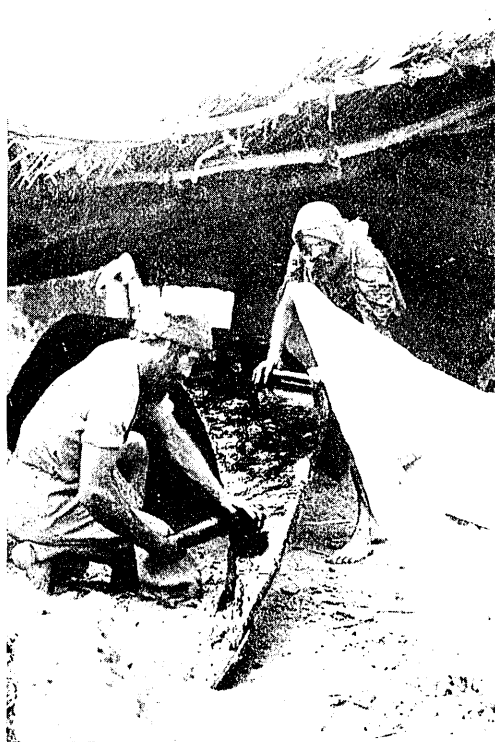
b. Şubbi boat-builders pitching a boat
