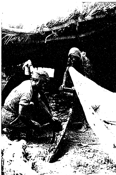
b. Şubbi boat-builders pitching a boat
