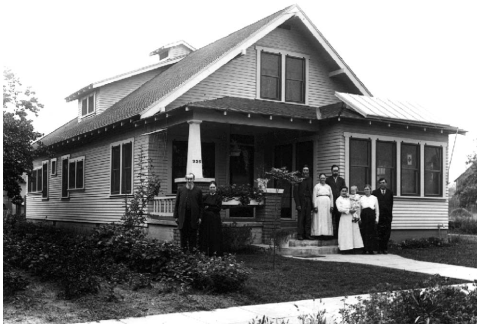
FIGURE 7 An early flat plate collector installation. From Perlin/Butti Solar Archives.
