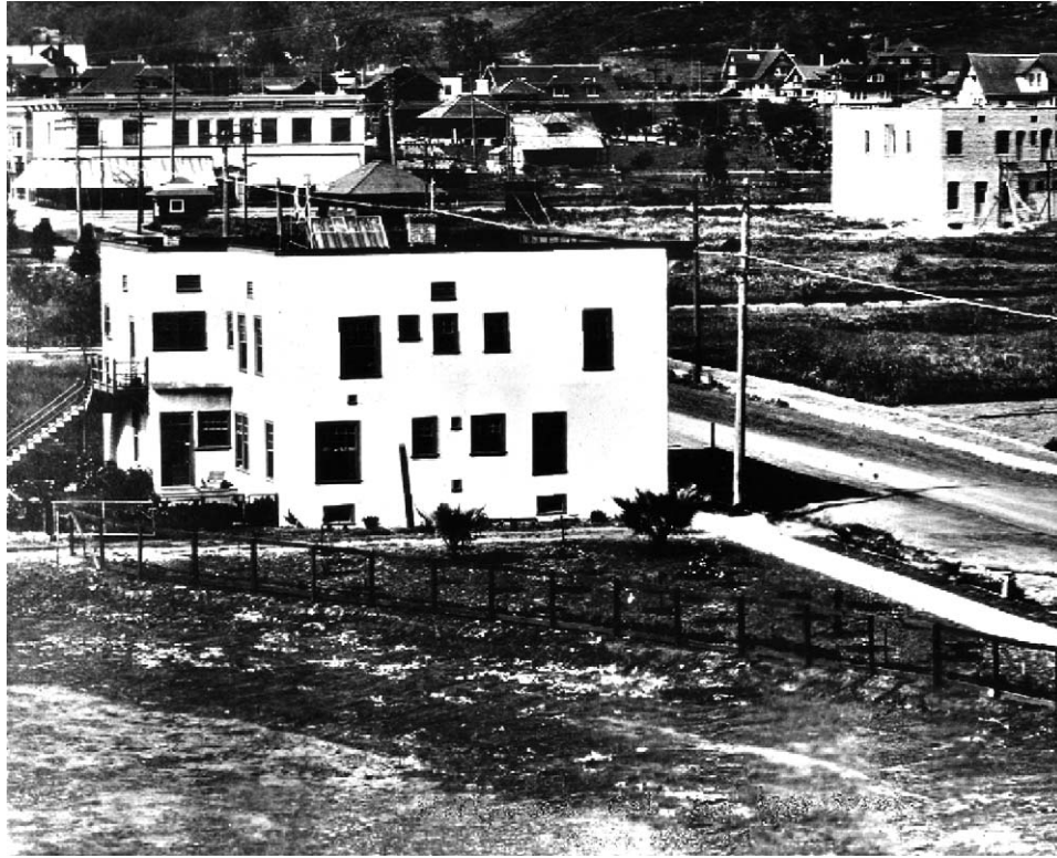
FIGURE 5 Installation of tanks in glass-covered box, Hollywood, California. From Perlin/Butti Solar Archives.
