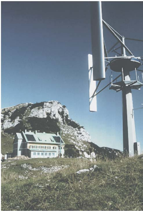
FIGURE 5 The Rotwand house in the German Alps. Electricity is provided with a PV, wind, and diesel hybrid system in operation since 1992.
