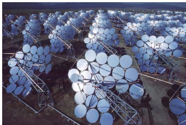
FIGURE 12 Seven hundred dishes producing steam for a central turbine system. Source: LaJet.
