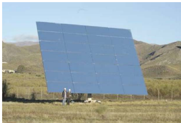
FIGURE 6 A 120 m 2 heliostat for central receiver power plants. Source: Sanlucar-120.
