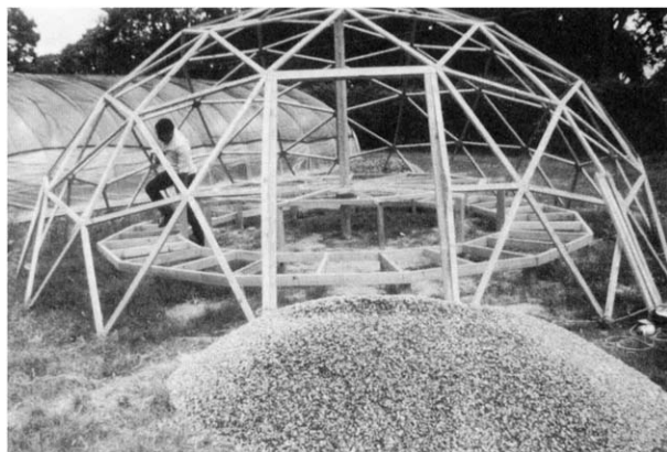
FIGURE 11 Structure of a geodesic dome dryer.
